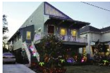
Julie: "My neighborhood has been reborn. Out of 22 houses located in my block, 16 were torn down. Of those, only three lots remain as blank slates for a new house. The rest have been rebuilt, including my own. It is a new old neighborhood."
